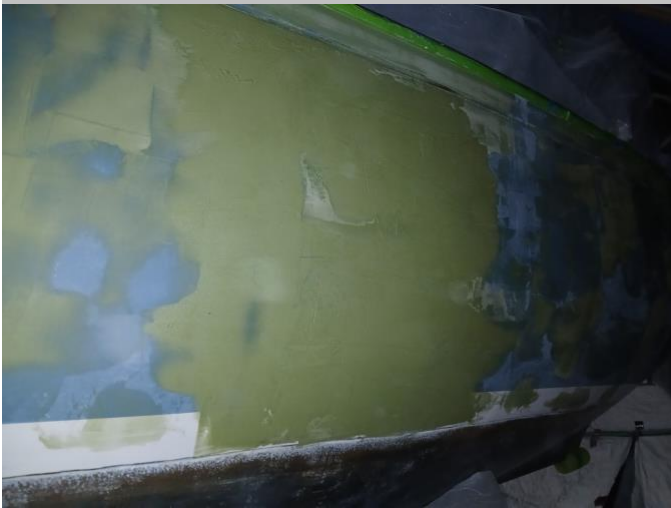
Figure 27: Newly faired areas damaged by previous attempts to repair.
