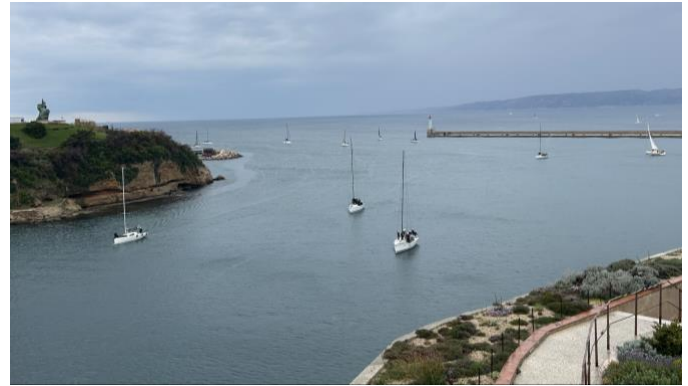
Figure 1: Looking SSE, harbor entrance.
