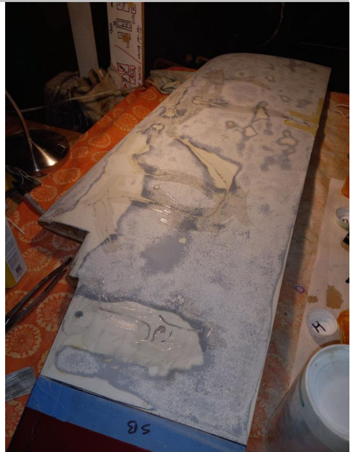
Figure 6: Below waterline cracks and pintle bracket holes filled with epoxy and ready to drill and sand.
