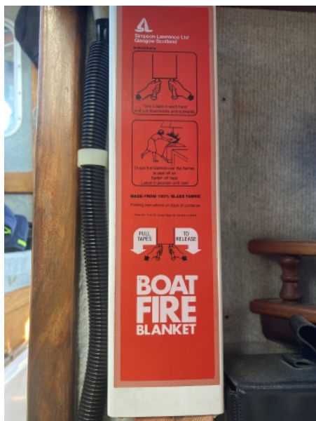
Photo 1: A fire blanket mounted to a boat bulkhead for easy access.
