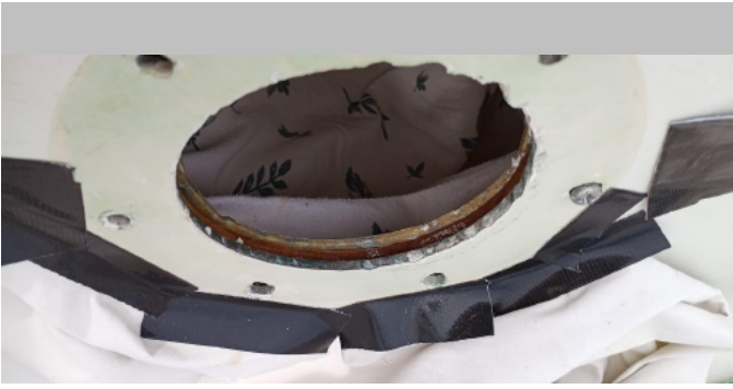
Photo 3: View from exterior looking down. Between the outer and inner walls you can see the edge of the insert in its final placement (slightly recessed and sandwiched between the outer wall and the interior wall).
