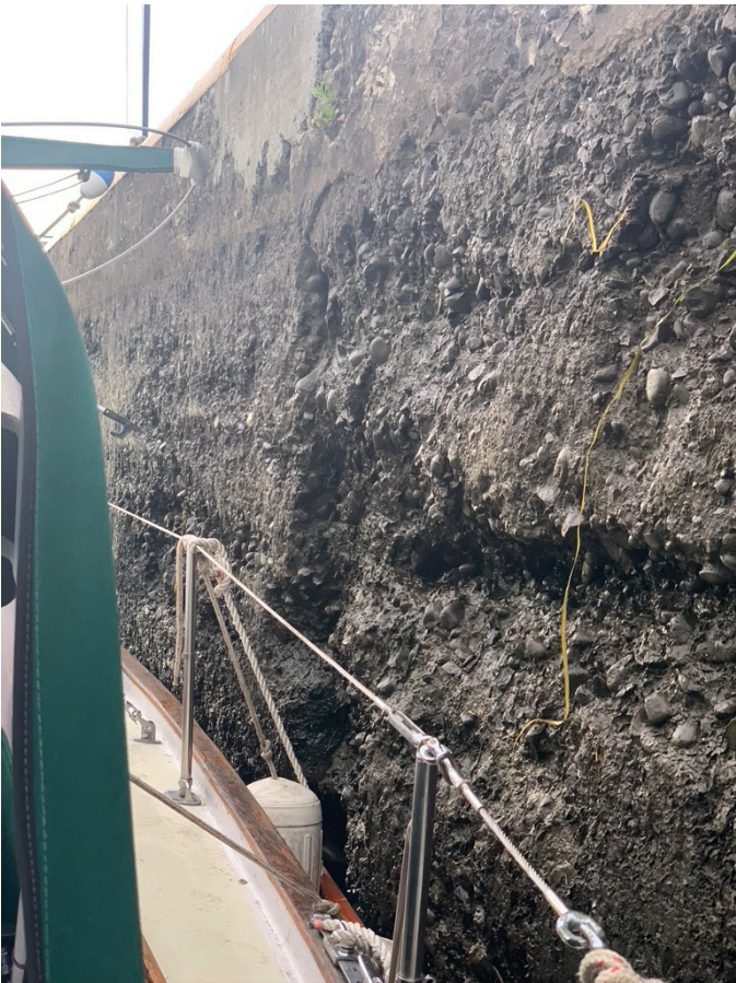
And here are the walls of Lock 15. I was worried that even our well-endowed fenders and fender boards wouldn't be enough to protect our hull.
