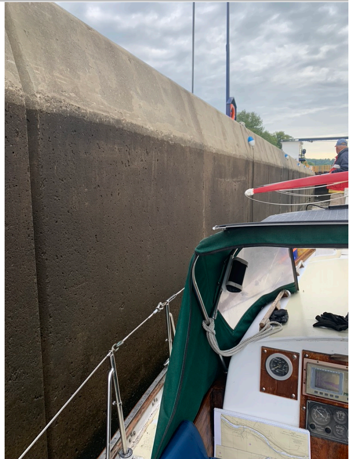
One lock later, at Canajoharie's Lock 14, we have some perfectly groomed concrete walls in the lock.
