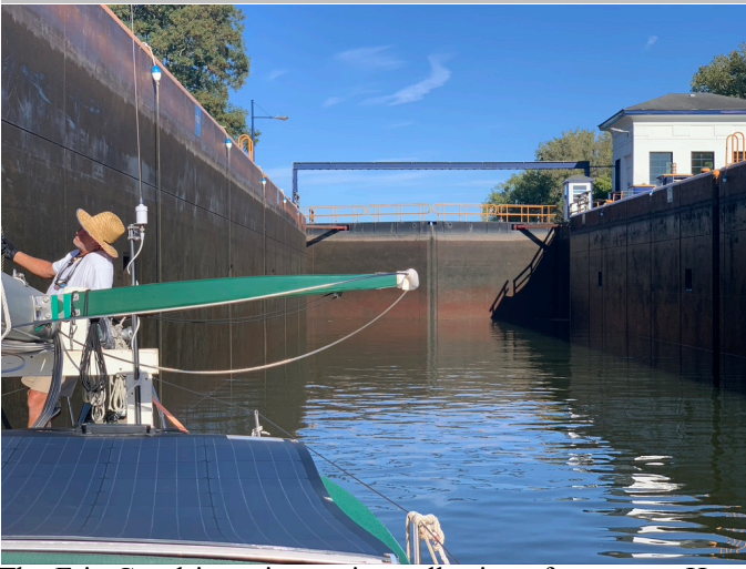
The Erie Canal is an interesting collection of contrasts. Here you see the very well maintained, steel-clad walls of Lock 16.
