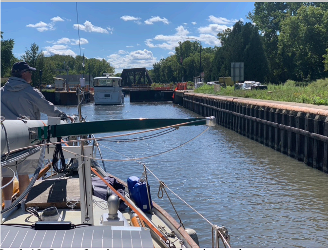
Lock 19: Lots of maintenance work going on here. As you can see, only the doors on the north side of the lock were functioning.
