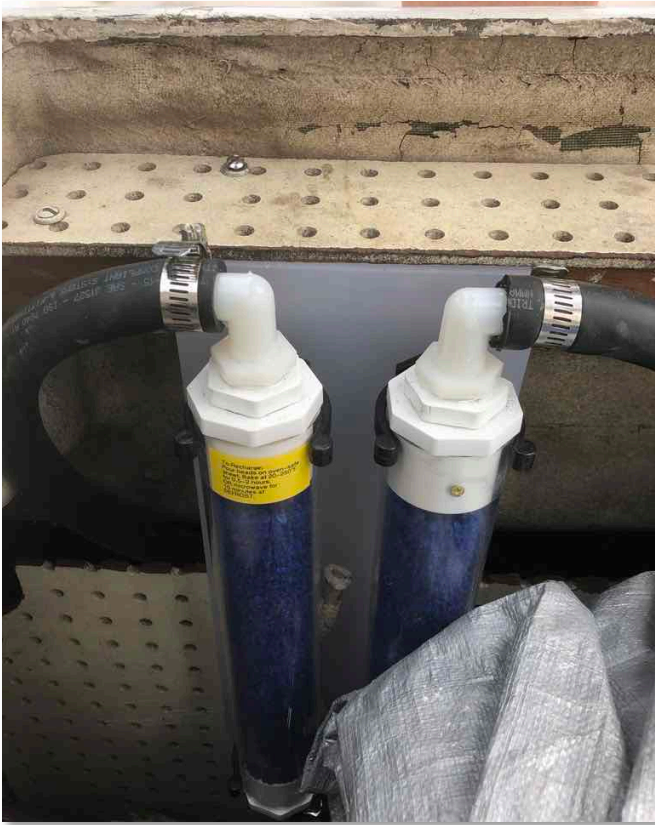
Photo 13: Final mounting location in the port cockpit locker.
