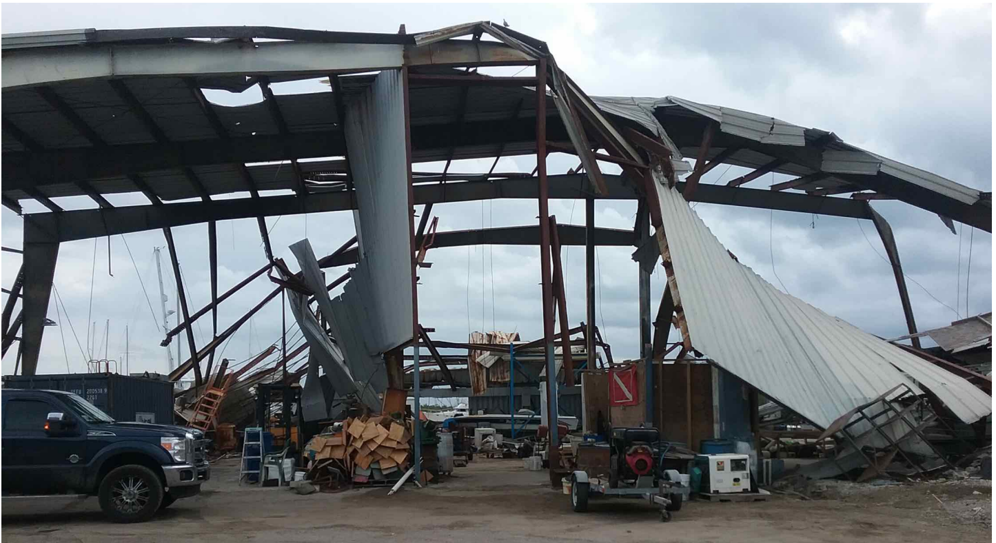
Photo 1: Main marina building - or what's left of it.
