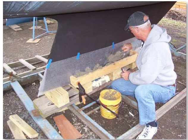
Figure 4 - Pouring the concrete to make the templates for the keel bulbs.
