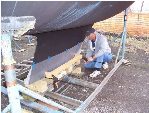
Figure 3 - Making the keel bulb molds.
