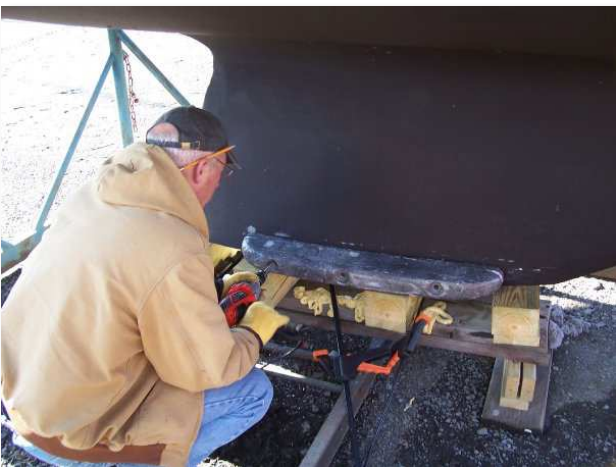
Figure 17 - Each bulb was attached with three 5/8-inch stainless lag bolts.
