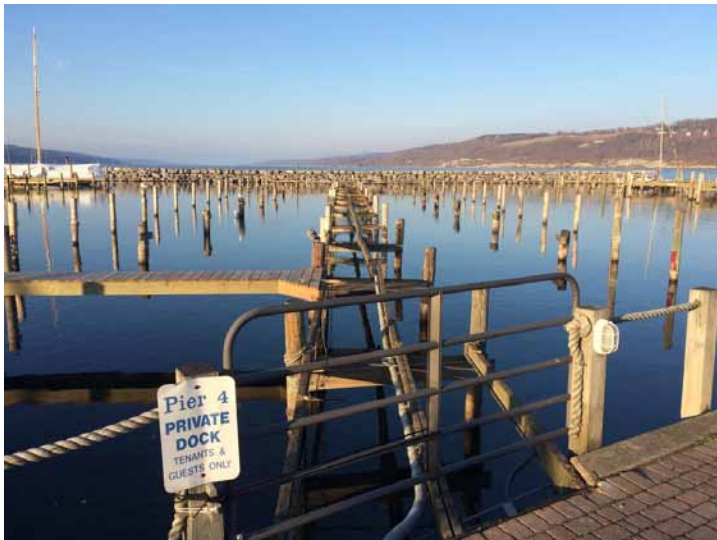
Pier 4 replacement was well underway in mid-November with nearly all of the old dock and fingers removed.
