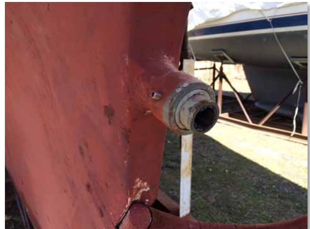
The cutlass bearing is held in place by a couple of Allen screws in a bronze collar around the stern tube. Removing the Allen screws allowed the collar to be removed and then the old cutlass bearing slid out rather easily.
